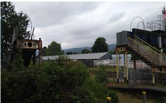
The lattice section of the footbridge has been removed and is now at our workshop in Cardiff
